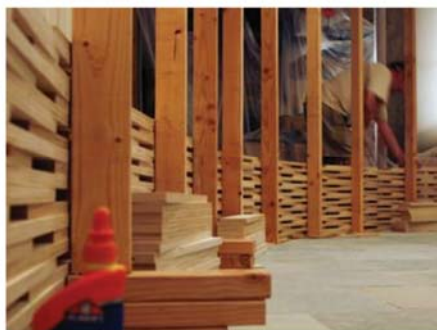
A model at left shows the way soft curves were used to streamline the space's awkward geometry and define activity areas. The Baltic birch planks were stacked like bricks to build the walls (below left), which were shored up with temporary braces (top right below) as building guides until completed. Interior walls, such as the one defining the guest bedroom below, are translucent.
